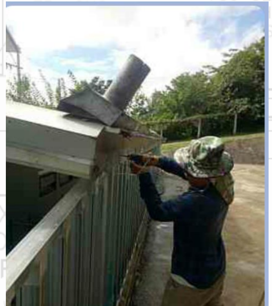
Fixing rain gutter for S2S
