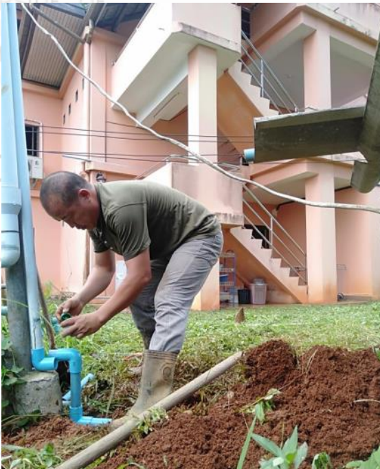
Fixing one of the main water pipes that was broken for Chiangrai YWAM Base
