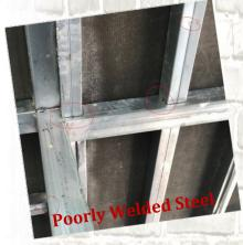
Once we got there, we met with the house parent. She walked us through the building and showed us where the problems were. The main issues we saw were poor welding on steel beams causing the house to become unstable to live in. We saw evidence of very little soil compaction on the location causing the erosion around the foundation of the building. We also did not see footings to support slab construction. This could cause a structural failure for the building.
